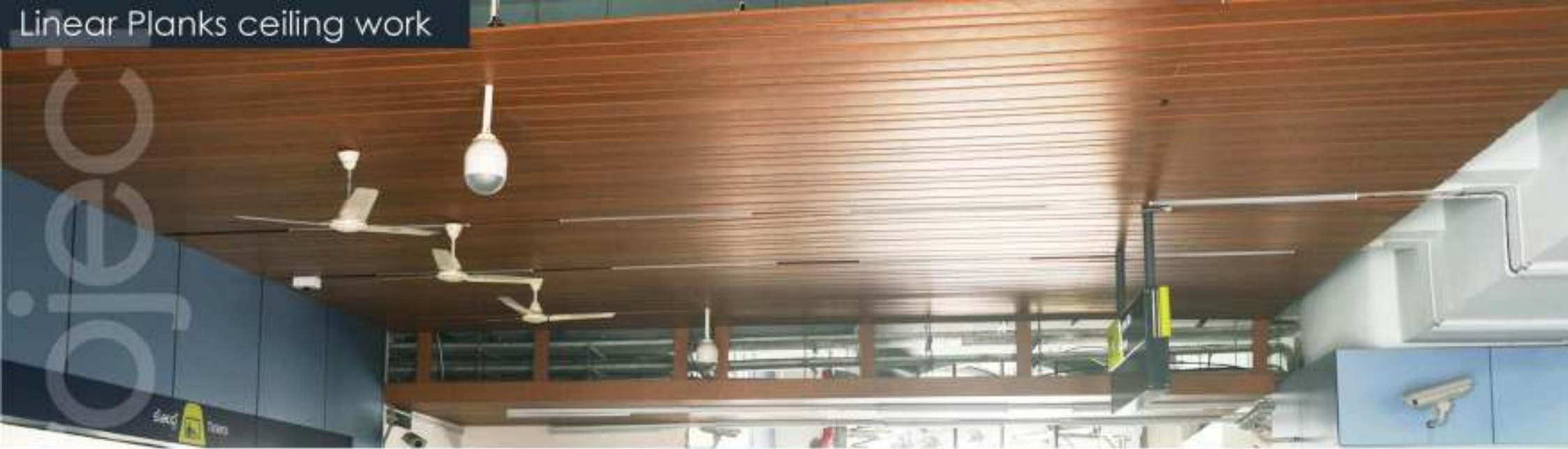
entrance portal work
